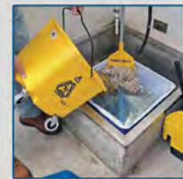
Mop Basin Drain Clogs
